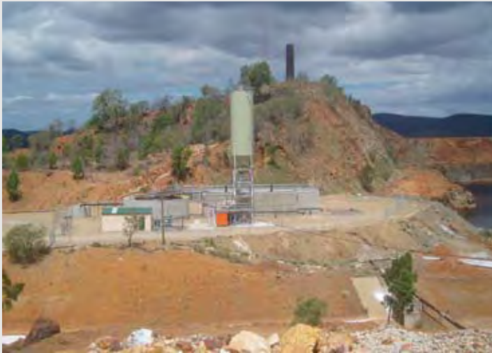
Figure 17: Pit water treatment plant adjacent to the AMD-filled open pit at Mt Morgan (March 2006)
