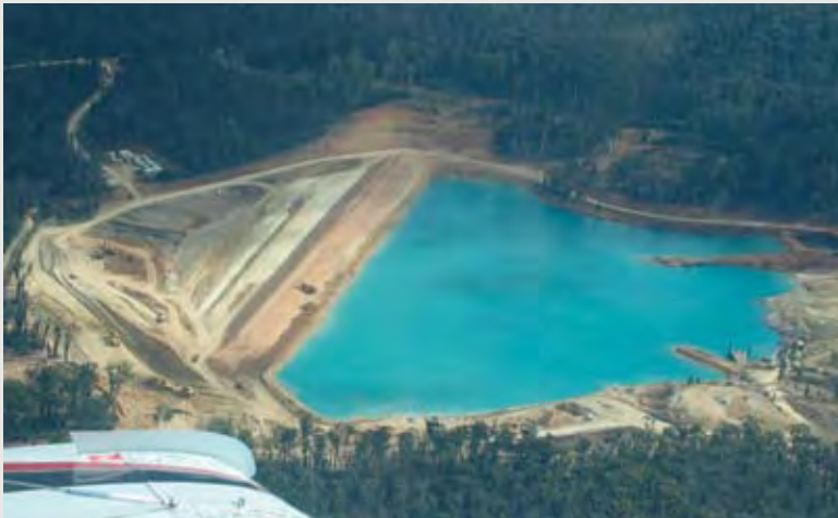
Figure 14: Aerial view of the Benambra tailings dam during rehabilitation works
