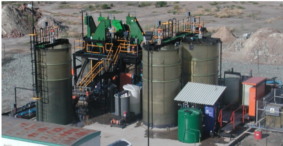
Figure 9: Demonstration plant installed on site at Harmony
