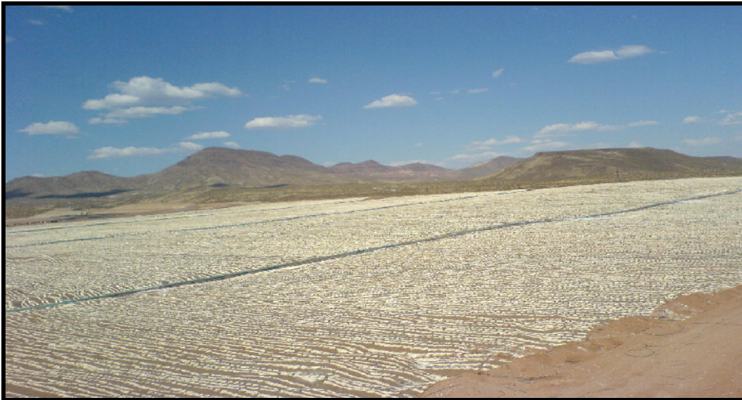
Figure 3.1 Copper heap leach pad.
