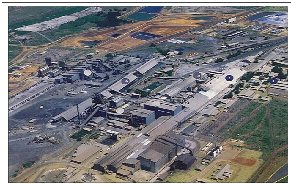
Figure 9: Middelburg Ferrochrome site
