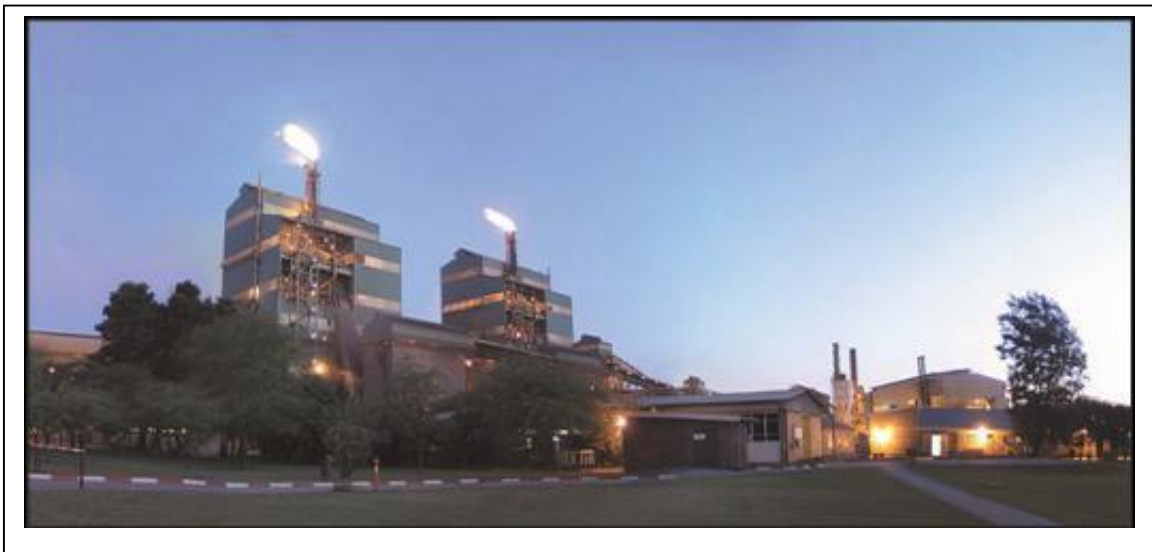
Figure 8: Furnaces F4 and F5 at Ferrometals
